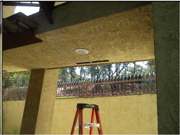
Typical Vent Opening
