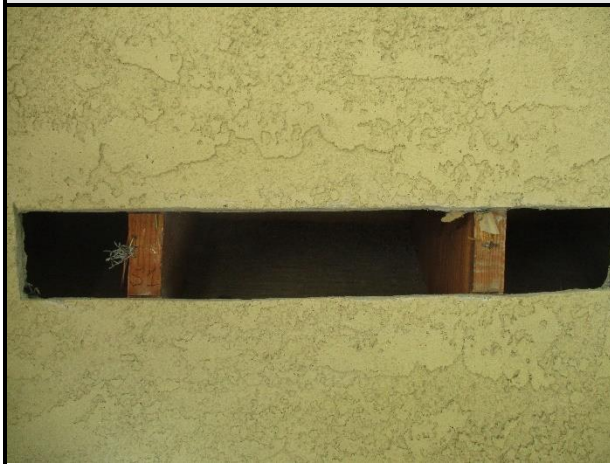
Inspection Vent at Stairs
