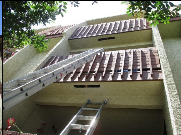
Typical Balcony View with Inspection Vents
